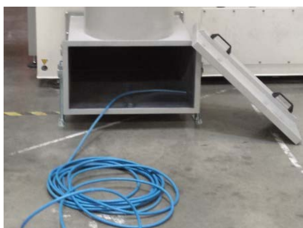
23. Clean the ducting
