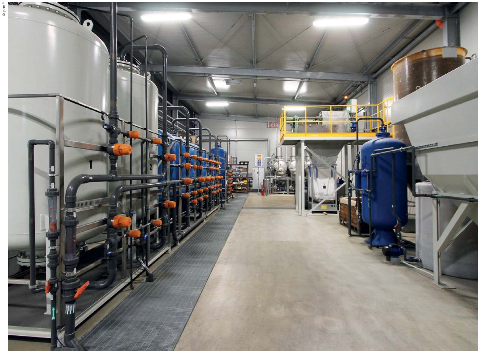
The zero-liquid discharge water treatment system and the demineralisation plant.
