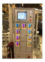
Gema CM30 control system. The state-of-the-art application system was combined with the reliable and still functional powder circuit, taking up very little space at all. Fresh and recycled powder are dosed via the ultrasonic sieve integrated into the monocyclone.
